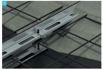
Place reinforcement and pour concrete evenly to both sides of the expansion joint at the same time. Finish surface and ensure top of joint is clear of any concrete.
