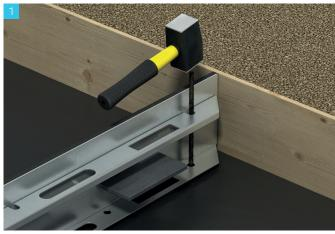
Position the expansion joint profile in the desired location and drive in the supplied pegs. Ensure the top of the peg is at least 20mm below the joint top.
