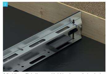
Adjust the profile to the correct height and secure by tapping in the supplied wedges and clamps  $\,$
