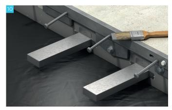
Apply bond breaker to the exposed face of the slab prior to placement of concrete for the second pour. The application of bond breaker to the existing face is important to prevent bonding of new concrete to existing concrete.
