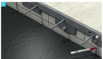
Mark drill hole locations at the specified centres for the post installation of the dowels to be used with Connolly Flange Dowel Box (FDB).
