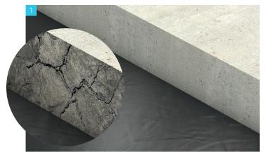
Prepare the existing slab for installation of Isedio Dynamic Extend profile by ensuring the face of the slab is straight, flat and the top and front is free from loose debris.
