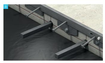
Inject Fischer FIS V 360 S epoxy into the clean drilled holes up to  $^2$ /3rd the hole depth and insert the dowel into the hole. Ensure the dowels are perpendicular to the face of the slab. Refer to epoxy manufacturer's installation guidelines for detailed information.
